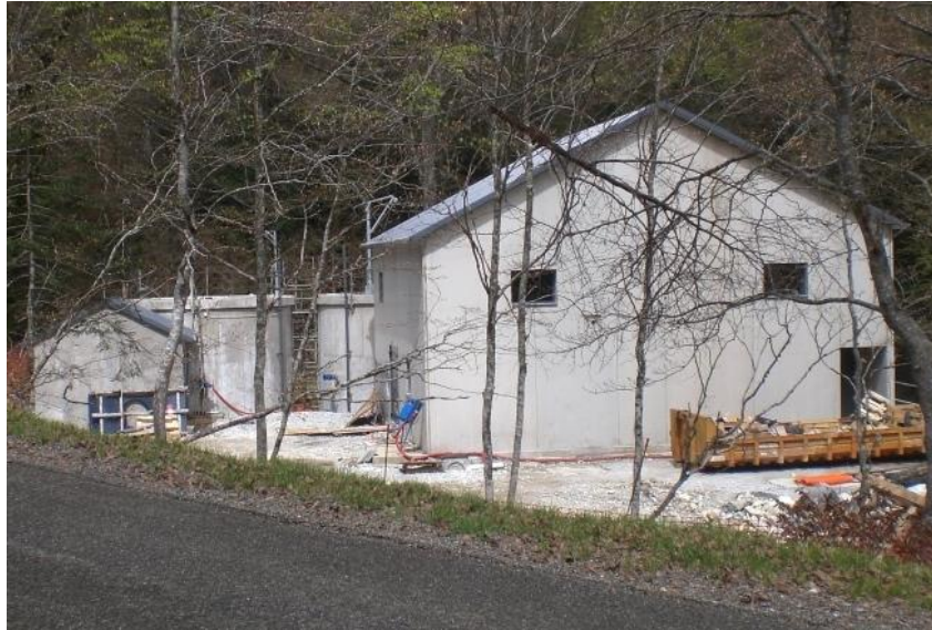
Figure 4: Example of SMBF plant in touristic site (5.000 PE)
